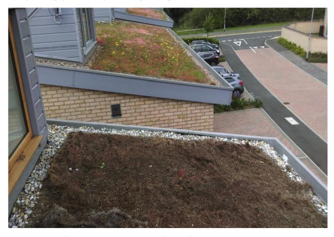
An extensive green roof destroyed by leatherjackets eating the fine roots of the Sedum and birds pecking at the blanket to expose and eat the Leatherjackets.
