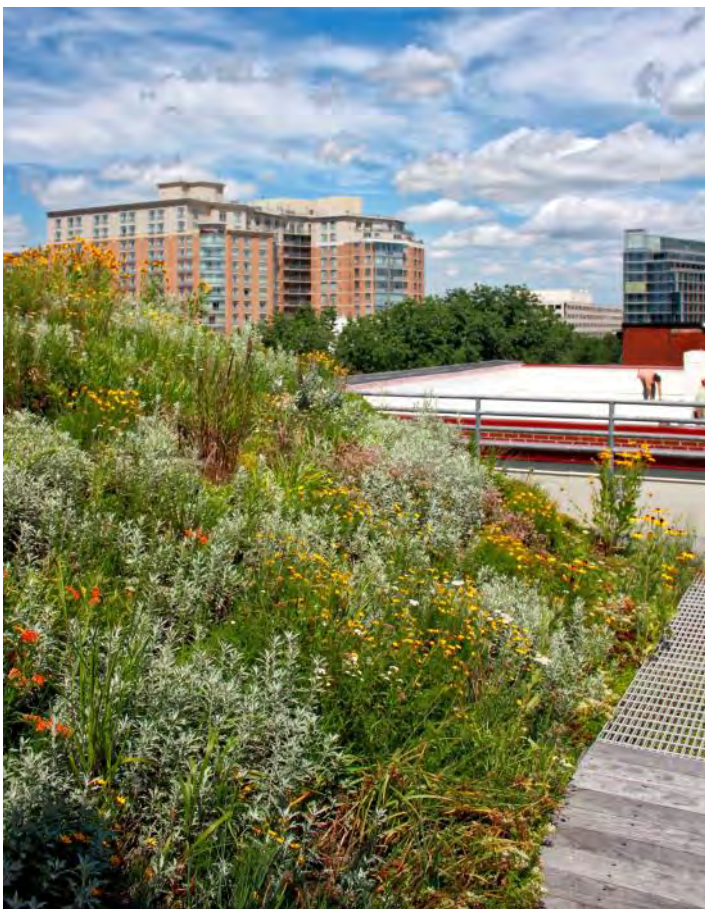
Extensive green roof, Washington, DC, USA.
