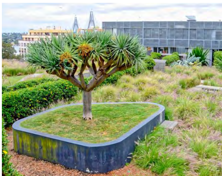
Intensive green roof, Sydney Photo: Matt Dillon
